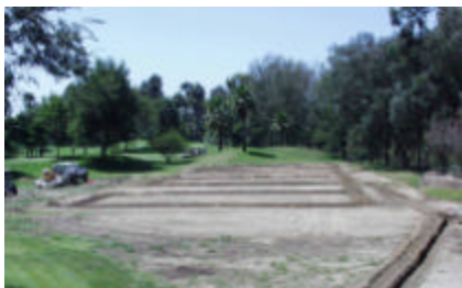
Trenching prior to irrigation system installation, 8/22/00
